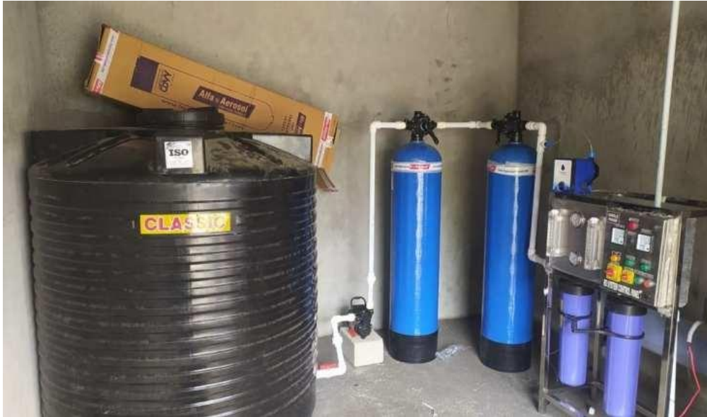
RO Water Plant at the time of Installation
